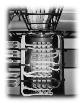
FIGURE 18.3 Lucent SYSTIMAX GigaSPEED Installation, rear view of patch-panel rack. (Copyright © 1999, Lucent Technologies, used by permission.)
